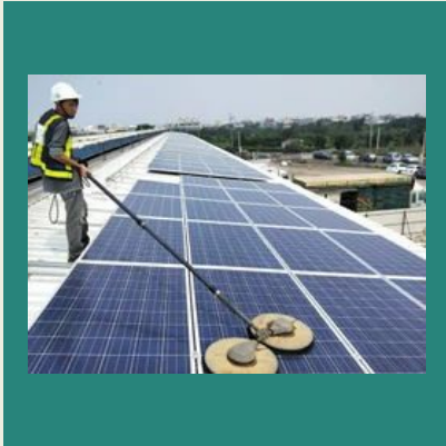
Solar Panel Cleaning
